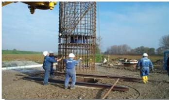
Installation of pile cage with O-cell assembly
