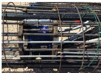
O-cell placed 2 m from the bottom of a Ø1200mm pile, mobilising 18MN
